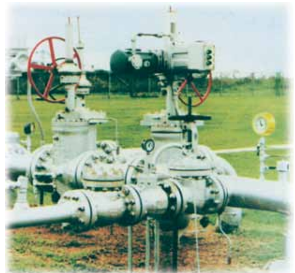
M&J Valve surge relief system protects pipelines from transient pressure surges
