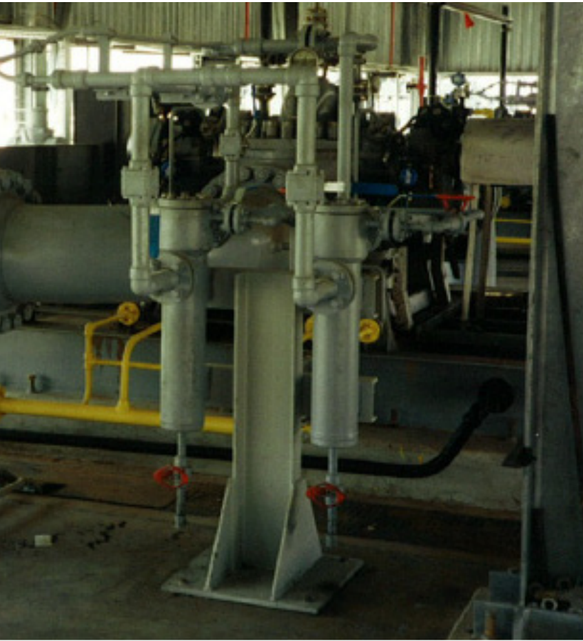
Image left: Improved filtration system for mechanical seal
