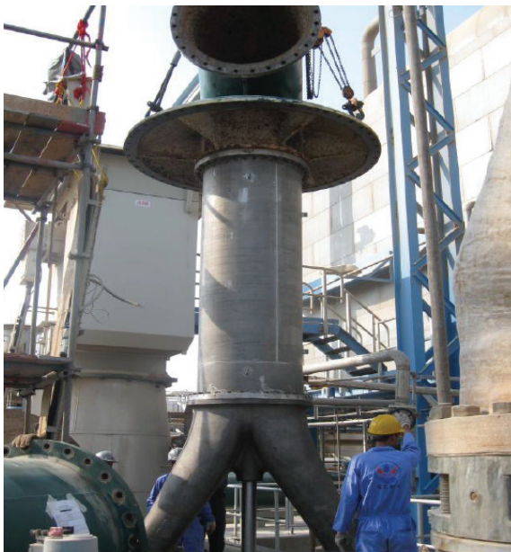
New casing being installed
